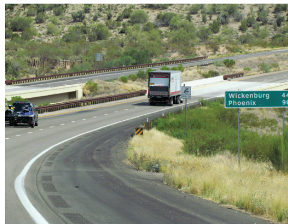
ADOT is improving US 93 to a 4-lane, divided highway between Wickenburg and the Nevada border, which will serve as an interim facility for I-11.
